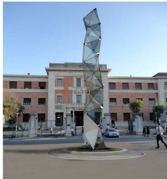
Fig. 2: Example of 15.00 meters tall HYGLASS installed at a roundabout in front of the School of Engineering main building (Pisa), taken from Froli and Laccone (2018)
