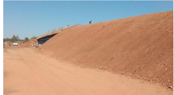
Fig. 2: Embankment of the level crossing at the Kossodo roundabout (Ouagadougou)
