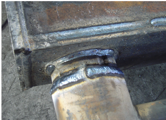
Fig. 6: Leg-pile connection joint, full-penetration weld of deck on top of piles
