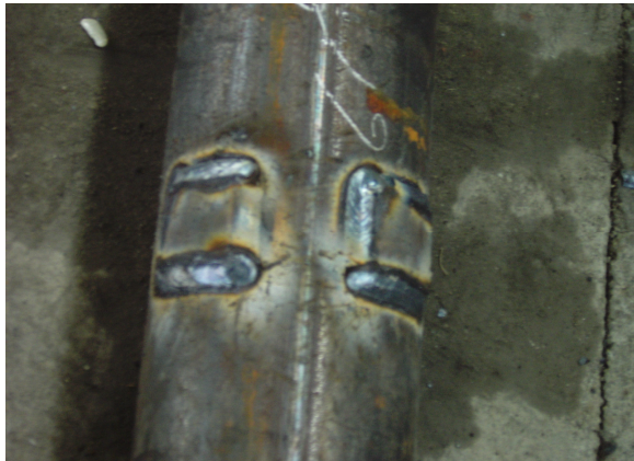
Fig. 5: Assemblage of shim plates on piles at mid-horizontal brace elevation
